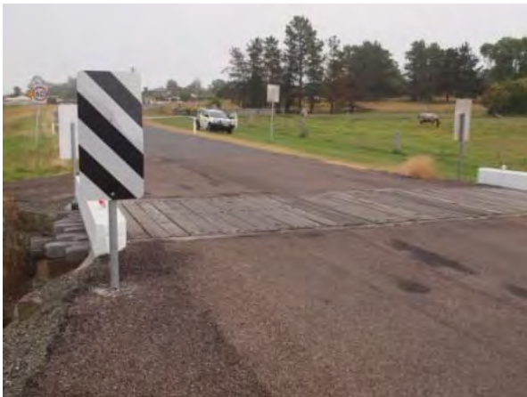
Branxton Road culvert, Greta (RPS 2016)
