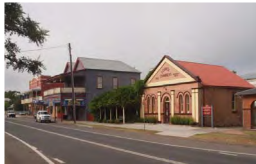
Plate 4: New England Highway – former Council Chambers (RPS 2016)
