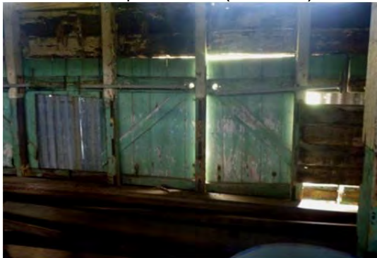
Byora – previous dairy shed, internal (RPS 2016)
